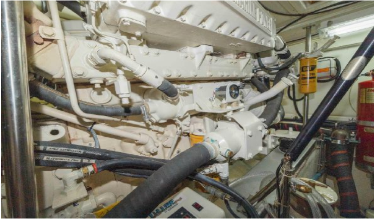
Well Maintained Port Engine
