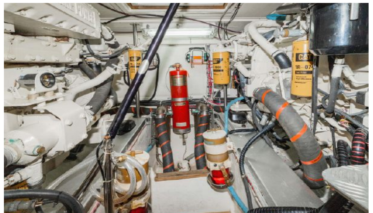
Well Maintained Engine Room
