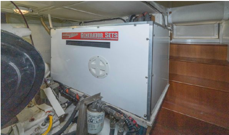
Northern Lights Generator
